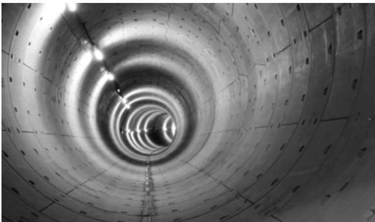
North-South METRO, Amsterdam
