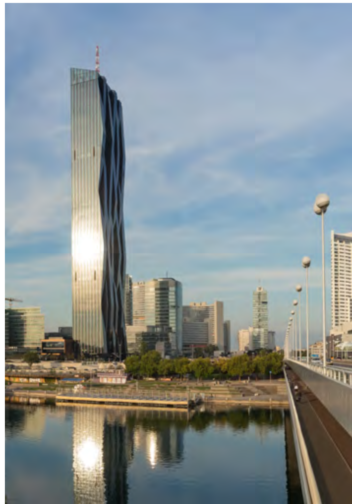
DC Tower 1 in Wien Foto: Hubertl
